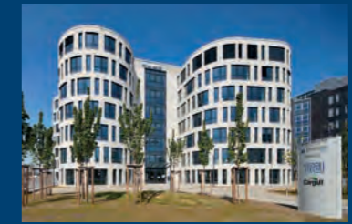
Relocation to a new office in the Airport City Düsseldorf 2020
